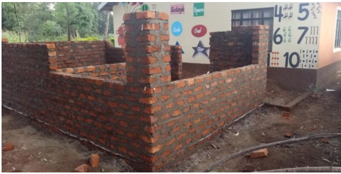
ECD new kitchen under construction.
