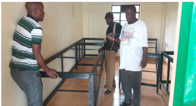
Science Lab Installation
