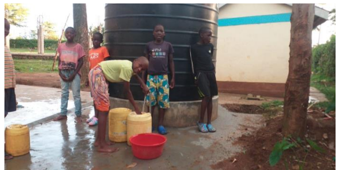
New water tank for boy's dormitory
