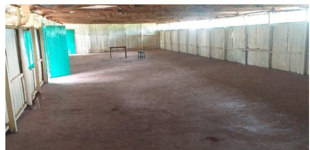
The old tin school building has been repaired and is now being used as a multi-purpose/dining room.
