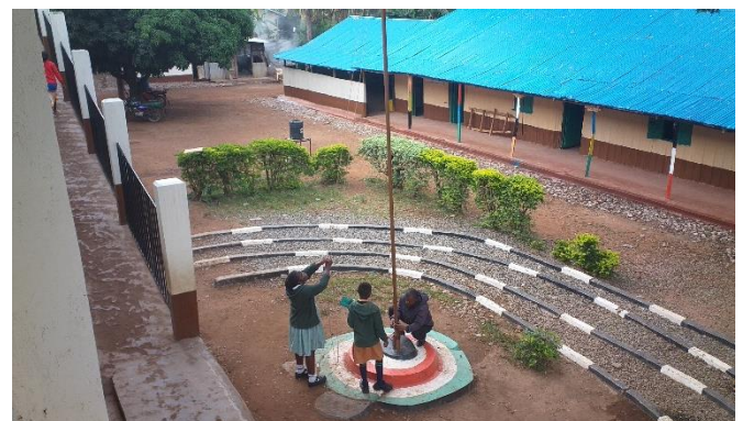
Area used for assembly has been repaired.
